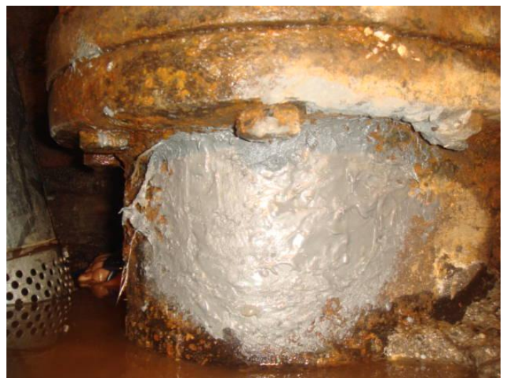
STEP 1: INITIAL COATING OF ECOPOWER'S COLD WELDING IS CARRIED OUT
