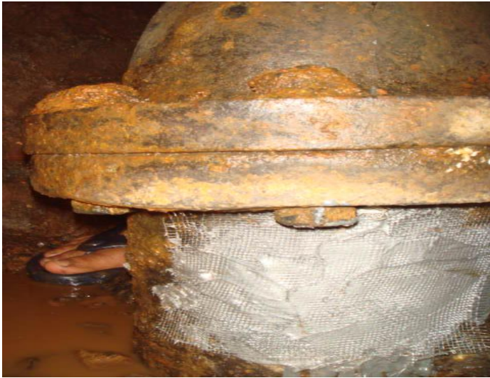
STEP 2: WIRE MESH IS PLACED OVER COLD WELDING COATING
