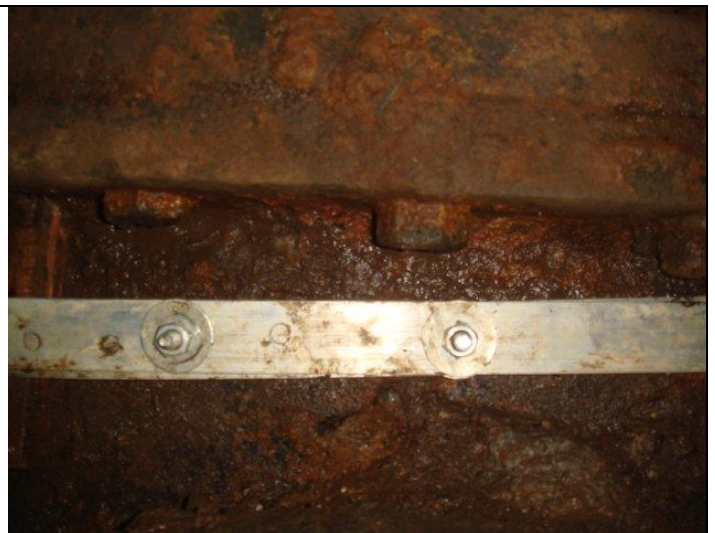
STEP 4 (B): ALUMINUM STRIP IS FASTENED FROM THE OPPOSITE END USING NUTS AND BOLTS
